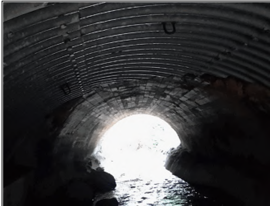
General View CMP and Concrete Arch
