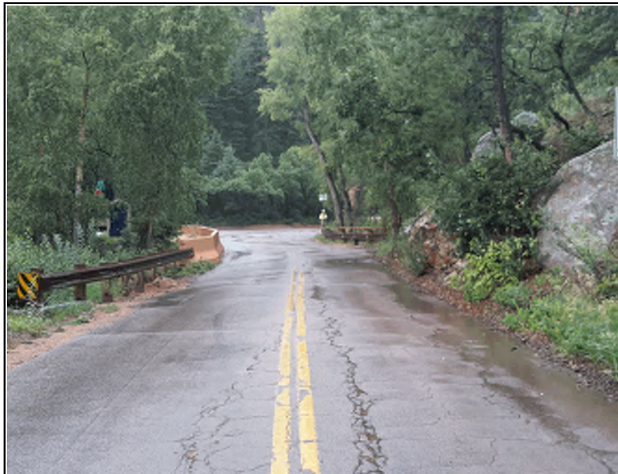
Approach Roadway Looking South
