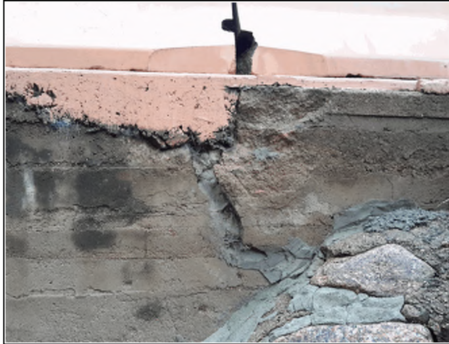
Cracking in downstream headwall has been repaired
