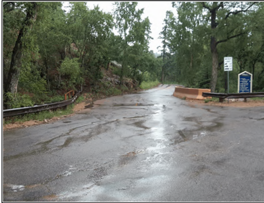
Approach Roadway Looking North
