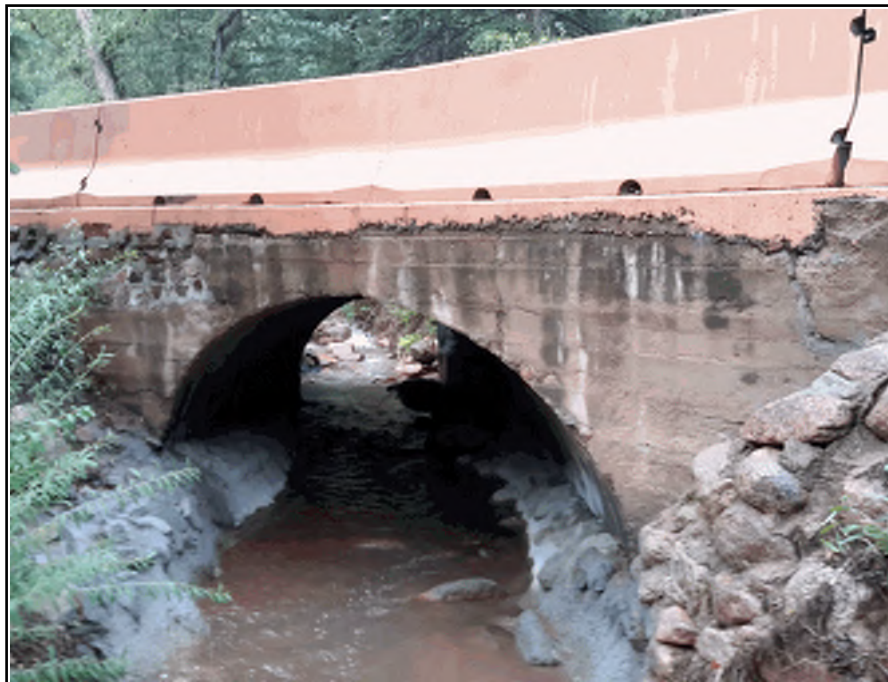
Downstream Elevation Looking West
