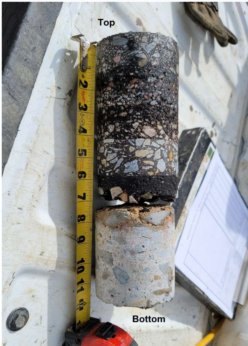
B-1 Pavement Core
