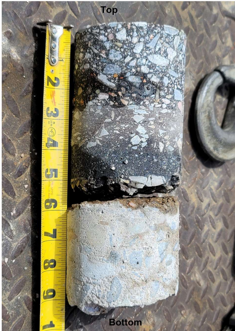
B-3 Pavement Core
