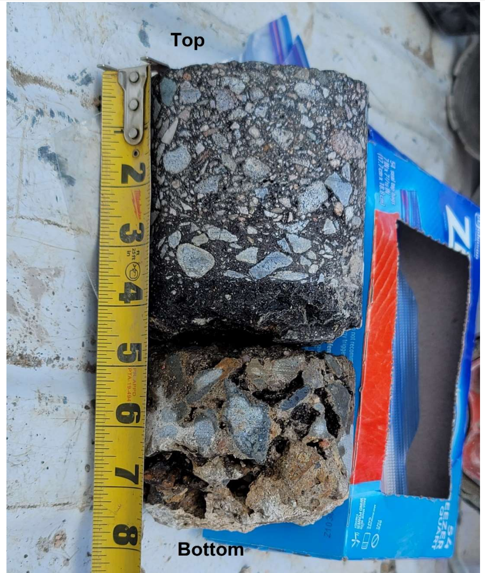
B-4 Pavement Core
