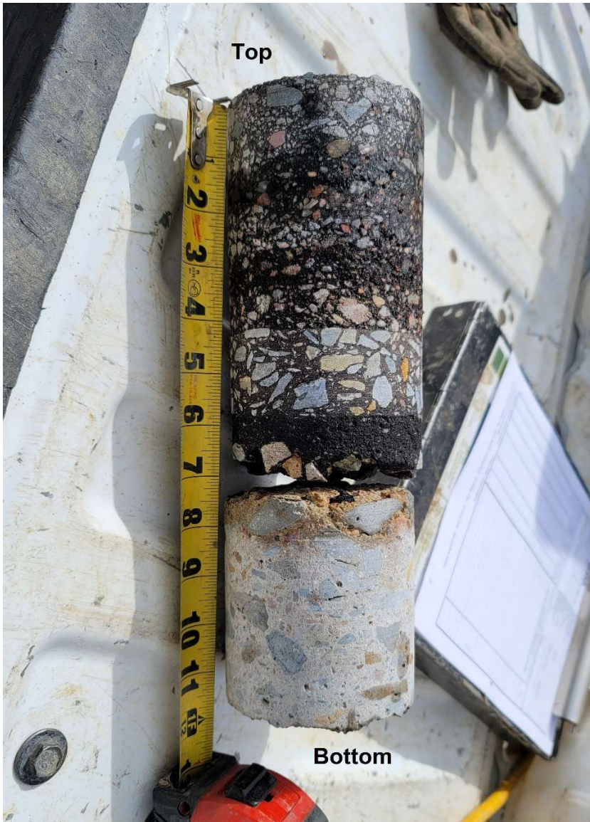
B-1 Pavement Core
