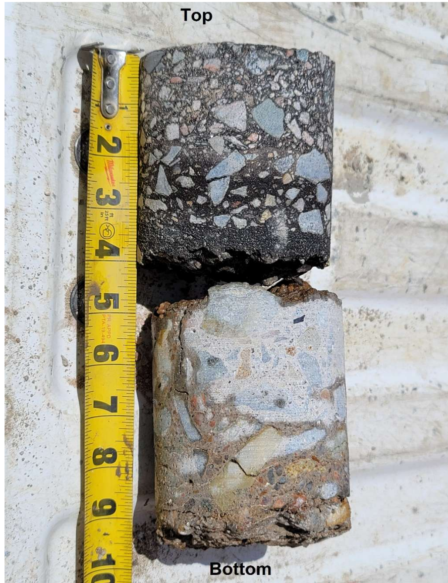
B-5 Pavement Core
