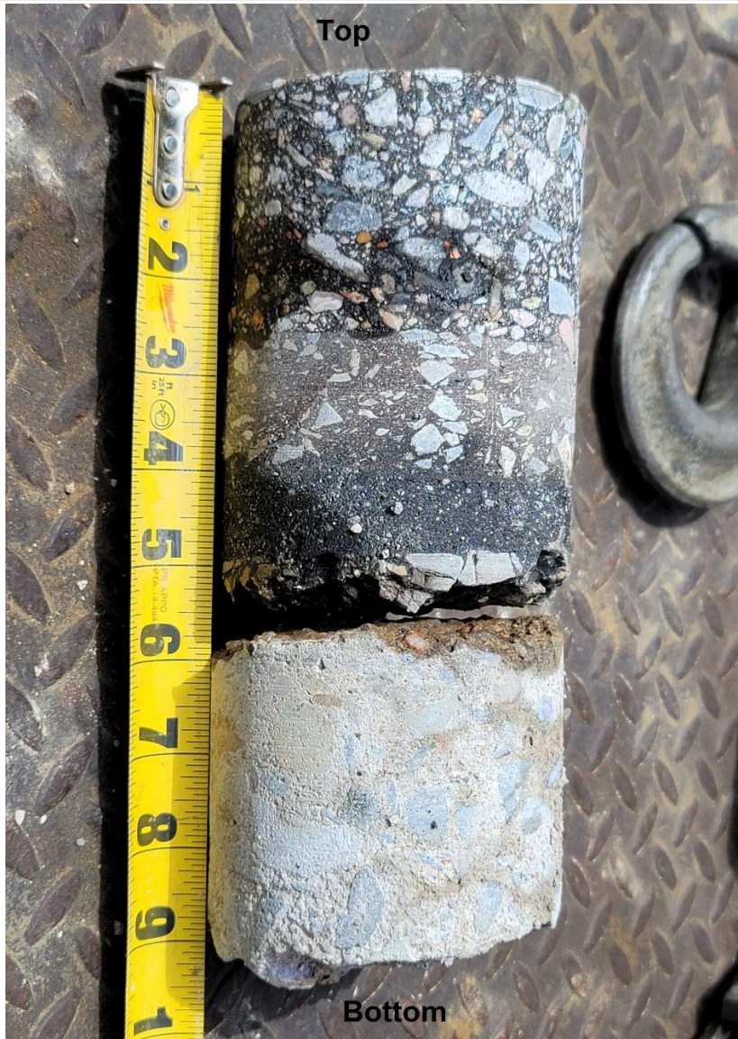
B-3 Pavement Core
