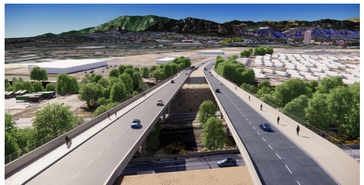
Above: a rendering of the completed project with new bridges, pedestrian and bicycle access.
