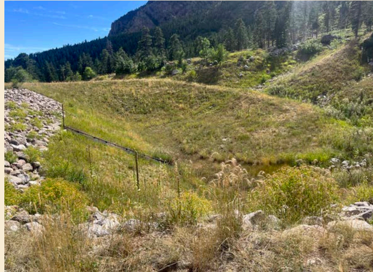
One of the debris basins within Fishers Canyon Open Space.
